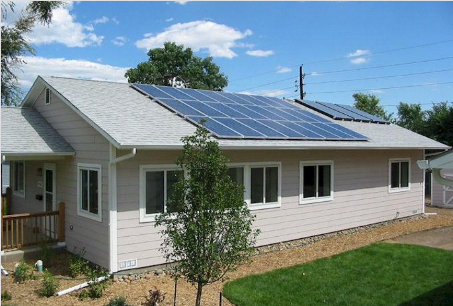
NREL's Zero Energy Habitat for Humanity Home: A Model for the Future of Affordable Housing
