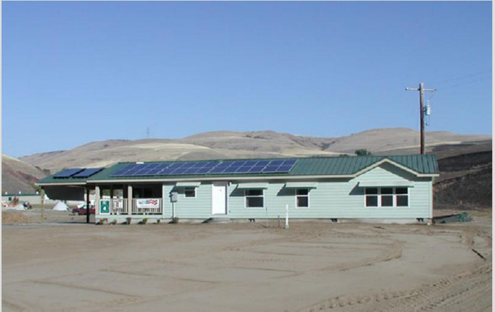
Nez Perce Zero Energy Manufactured Home Project
