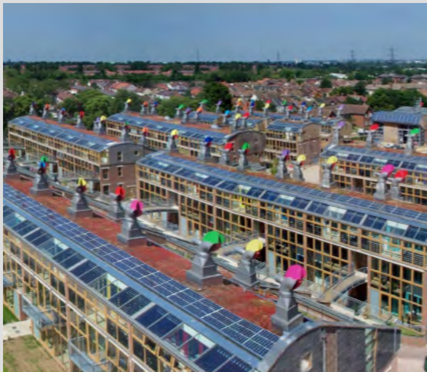
BEDZED zero-energy community (UK)
